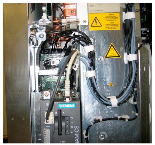
Figure 3-58 Mounting the CU310 in the Power Module chassis format, frame size FX
